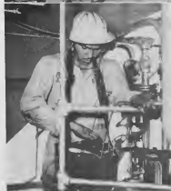
VICTOR THOMP, engineering assistant A, top left and above left, visually checks the inside of a gate valve and uses a depth gauge to measure wall thickness loss on a pipe. Employing an on-stream inspection technique, top right, is R. Gil who is testing corrosion agent in a product. At left and right are L. Giel and C. Polak, EIG inspectors, who are measuring shell and pipe thicknesses with Audigage, left, and Penetron, right.
